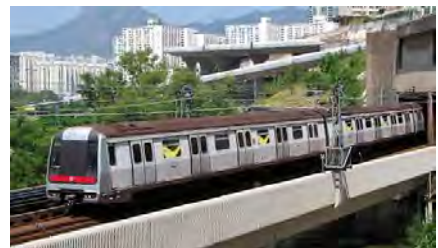
CCCR, South Island Line à Hong Kong
